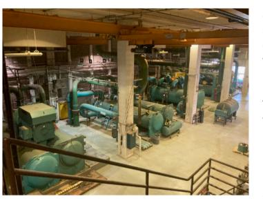
UTA's thermal energy production is a combination of two separate plants. The main Thermal Energy Plant (TEP) is located between the Health Center and Arlington Hall and this plant provides chilled water and steam various campus buildings. There is a second plant located behind the
