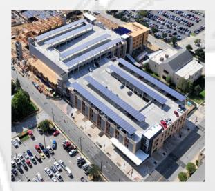
UTA designed and installed a 385 kW Photovoltaic system that became operational in 2011. This system is installed at the North Parking Garage Sections A and B. This location was selected for the large area and existing structure could support the added weight. The system consists of 1652 Schott 235 photovoltaic panels and two Satcon S-Type 210 kW inverters. Each panel is rated for 235 W max
